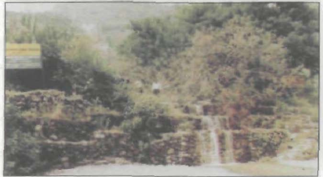
Stabilisation of limestone mine spoils
