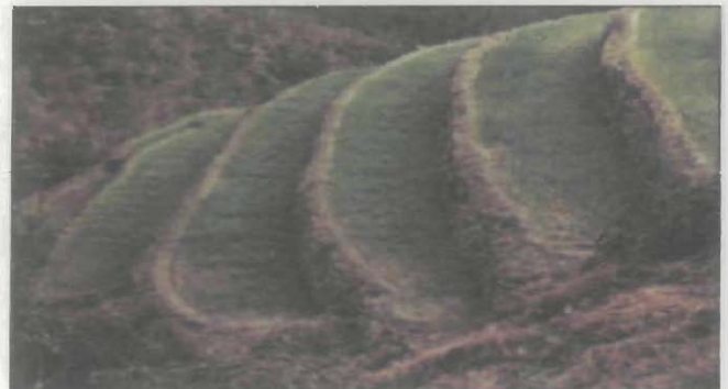
Bench terracing and contour bunding in mountainous watersheds
